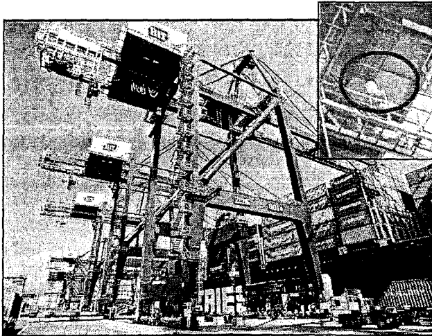
Figure 1. SaviTrak reader infrastructure on a quay crane in HIT terminal, Hong Kong.
