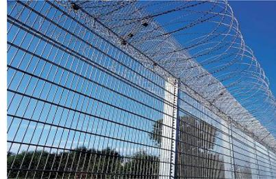
Razor wire can be installed above the barbed wire outriggers if additional security is desired. Steel posts can be set in concrete and bottom rails or tension wires can be installed at the base of the fabric. A trench at the base of the fence can be filled with concrete to prevent tunneling.
